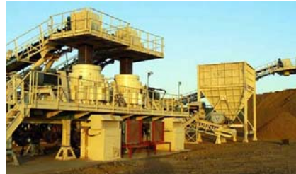
Crushing to -3mm
