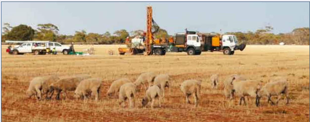
Figure 4 – YAJV Wheatbelt Drilling Operations.
