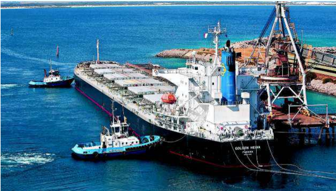
Fast track: The promise to expand the port to almost double its capacity would allow the Yilgarn province to grow
